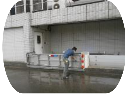
Flood response- Set up water-retaining gates
